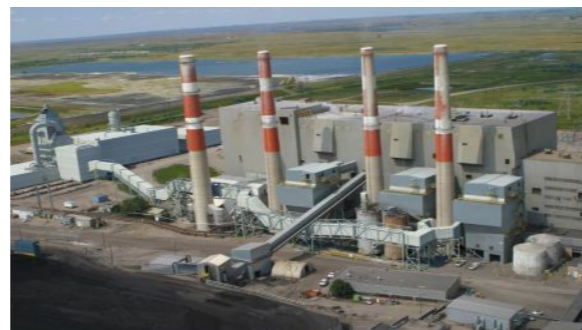
Boundary dam coal-fired power station
